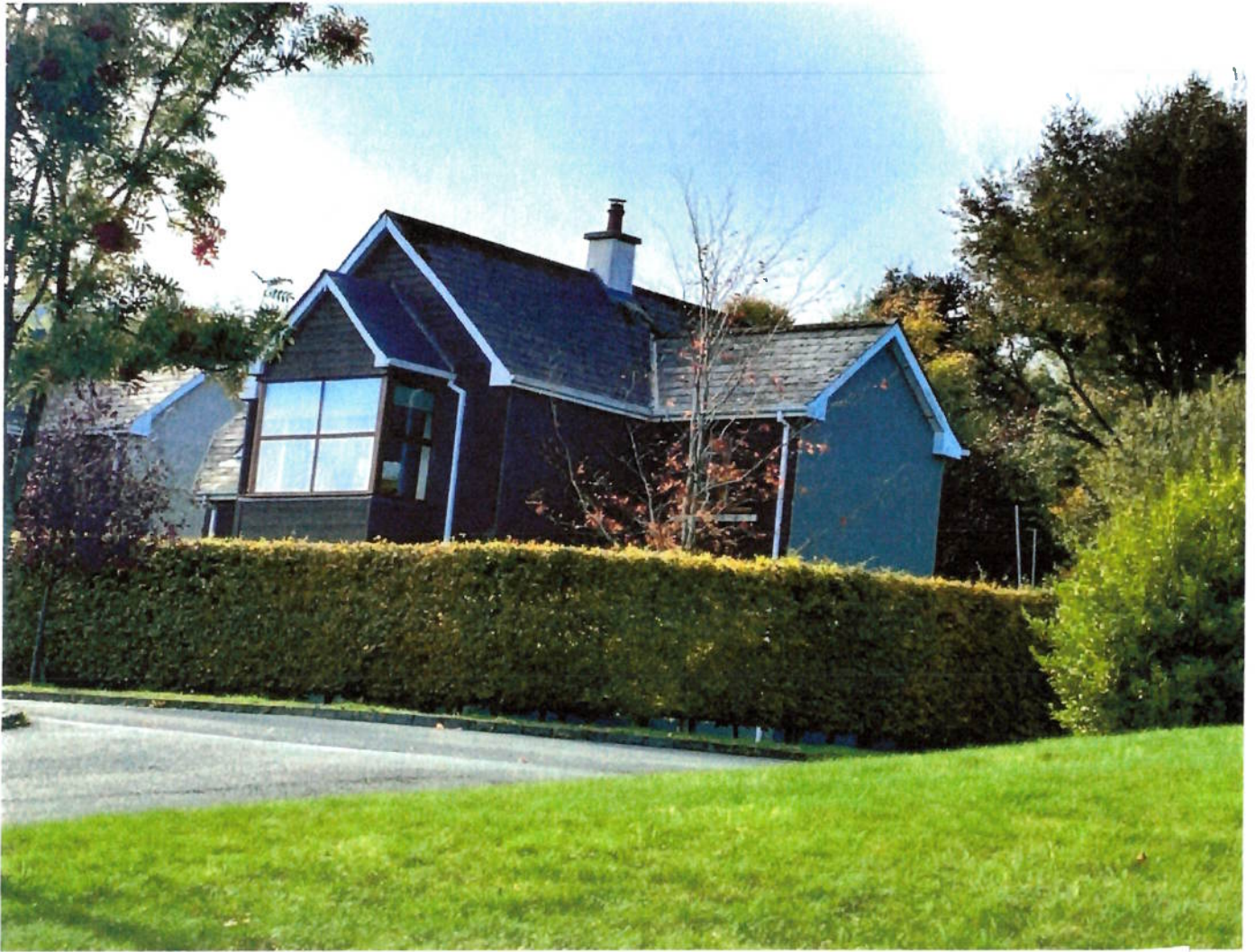
IMAGE INDICATING THE DETACHED DWELLING IN THE ESTATE WHICH HAS THE UPPER FLOOR BAY WINDOW BUT DOES NOT OVERLOOK A CLOSELY LOCATED NEIGHBOURING DWELLING AT A LOWER LEVEL
