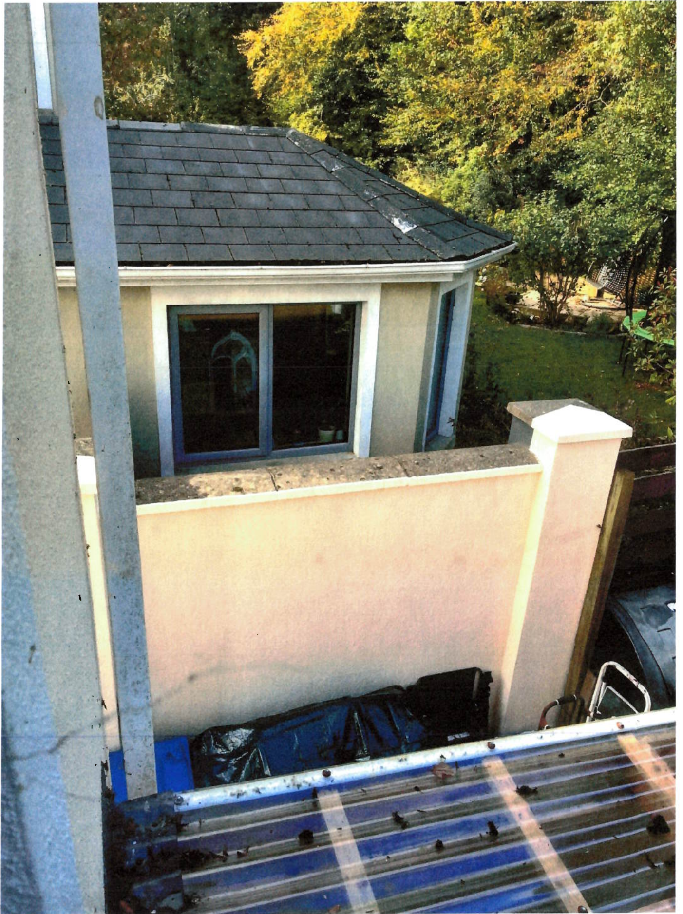
IMAGE INDICATING THE SUN ROOM CONSTRUCTED TO THE REAR OF NO. 10 BUT NOT SHOWN ON THE PLANS
